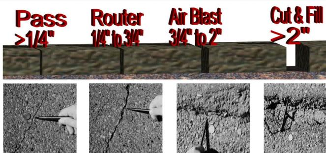
Graphical representations of typical crack sizes (from UFC 3-270-02)
