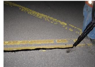
Crack Sealing Process
